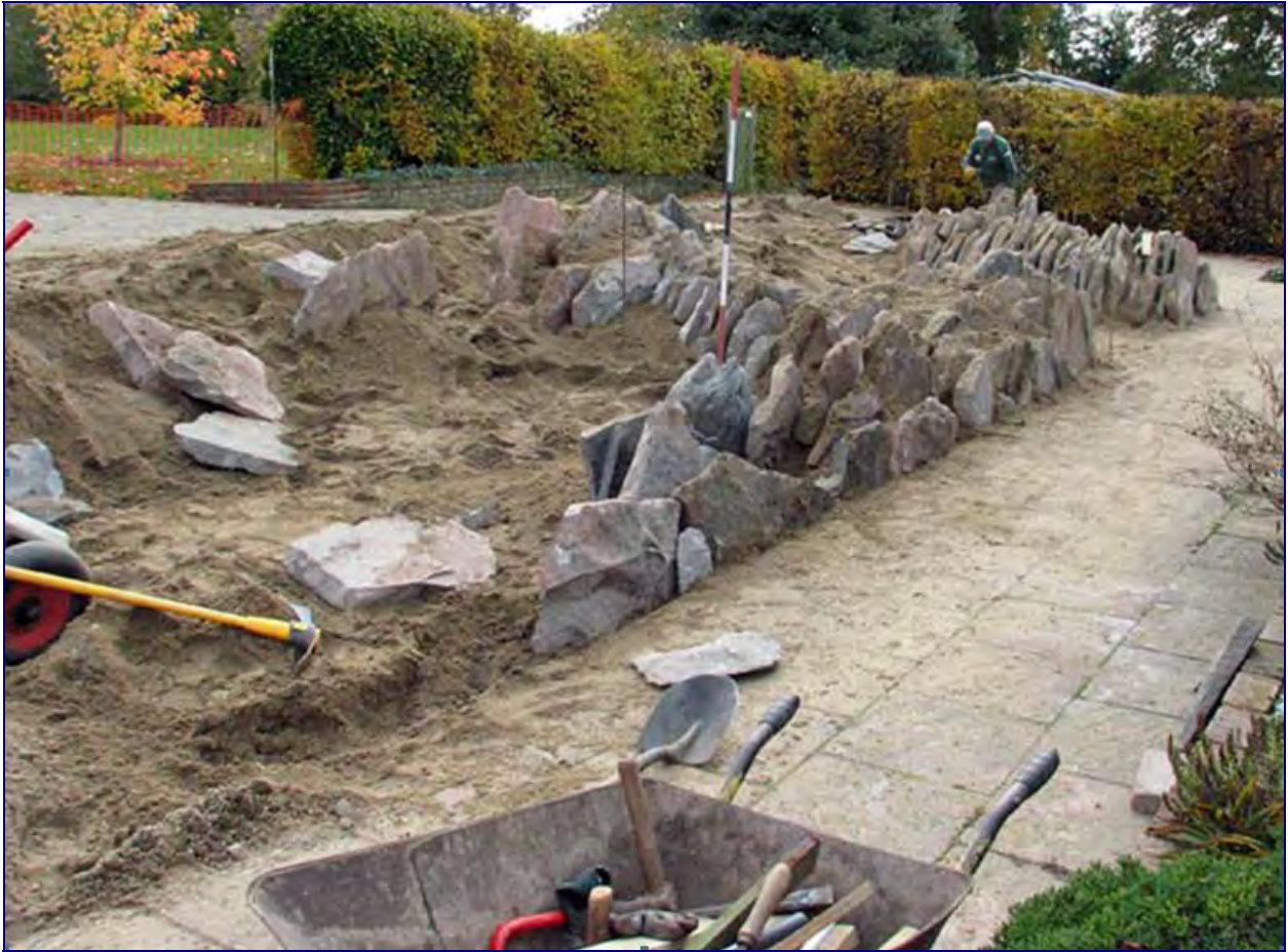
Above: The site during construction
