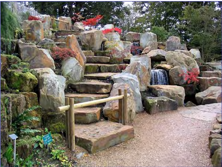
As it looked in October 2004 with the construction finished and some planting in place. The stone had been freshly quarried so looked very stark at first.
