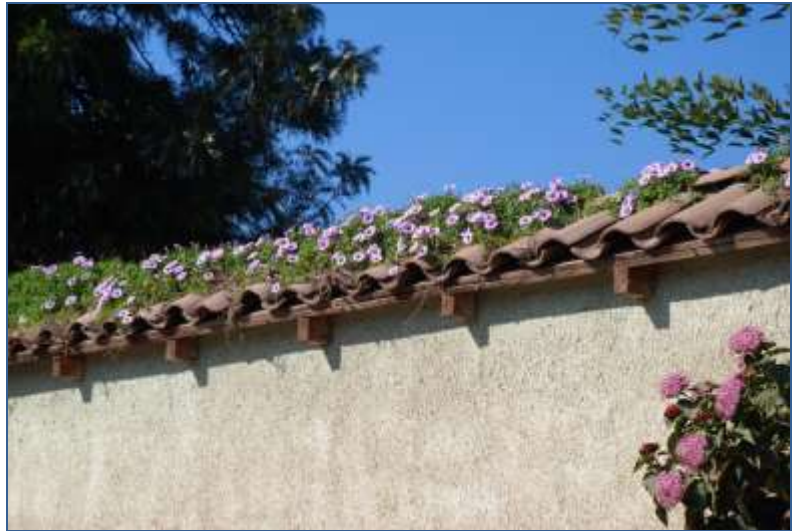
fig.60: Snap! The same Ipomoea cairica on our front wall at home in Chile. A view from the street. Note Clerodendron bungei , which has escaped out under the wall! (20 Apr 2017. JMW)
