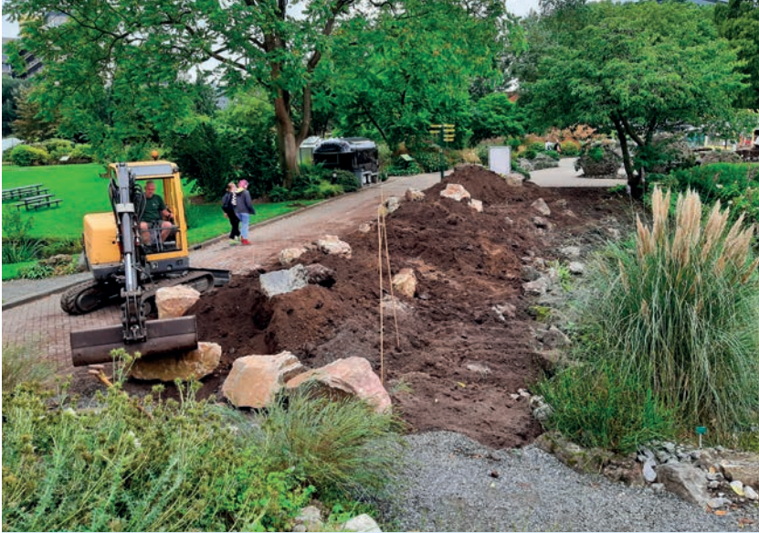
All stones are removed, soil moved into position, large rocks being placed
